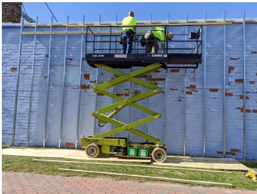
Al Kaikko and Brian Pence attach steel studs, which minimize warpage. Side benefit: The mural covers spalling paint.
